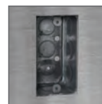
TA-62F Empty Junction Box
